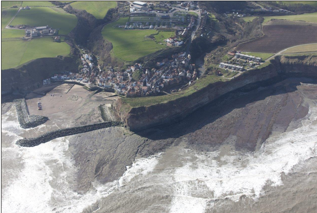
Figure 2.1. Location of Staithes harbour and Staithes village - east harbour arm is on the left of the images and west harbour arm is on the right of the image (Source: North East Coastal Observatory).
